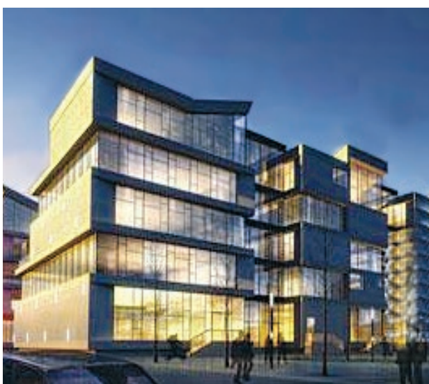
Intelligent commercial building, Shanghai
